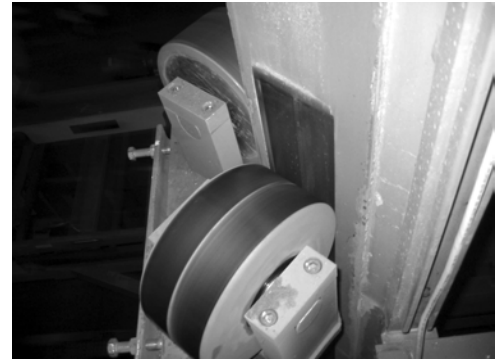
Floor-to-floor elevator guide wheel of NYTEC-HS
